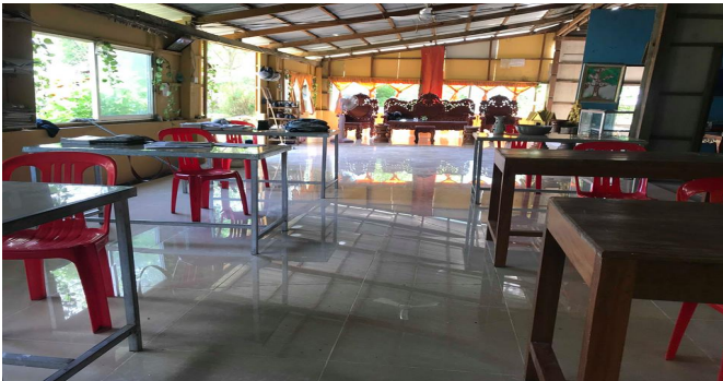
Flooring at Tampung Student Centre
