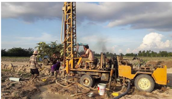
Sinking the borehole at CROAP, near Pursat
